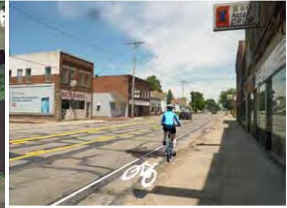
**Adaptation with Minor or Major Lane Modifications.** The 5th and 6th Street SW project is an example of a lane reduction, converting a lane that is not required for parking or traffic purposes into a bike lane. Other potential projects in this category include a cycle track over the Kentucky Avenue river bridge to link Birch Drive and the East Park Trail or a reduction of lanes on N Federal Avenue.
