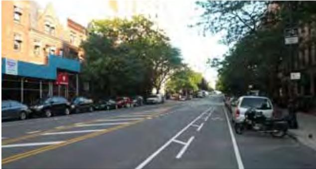
**Buffered bicycle lane.** Separation is provided by a cross-hatched neutral ground in this application in New York City. Some places use diagonal tick marks extending out from the parking lane line to mark the extent of the “door zone.”
