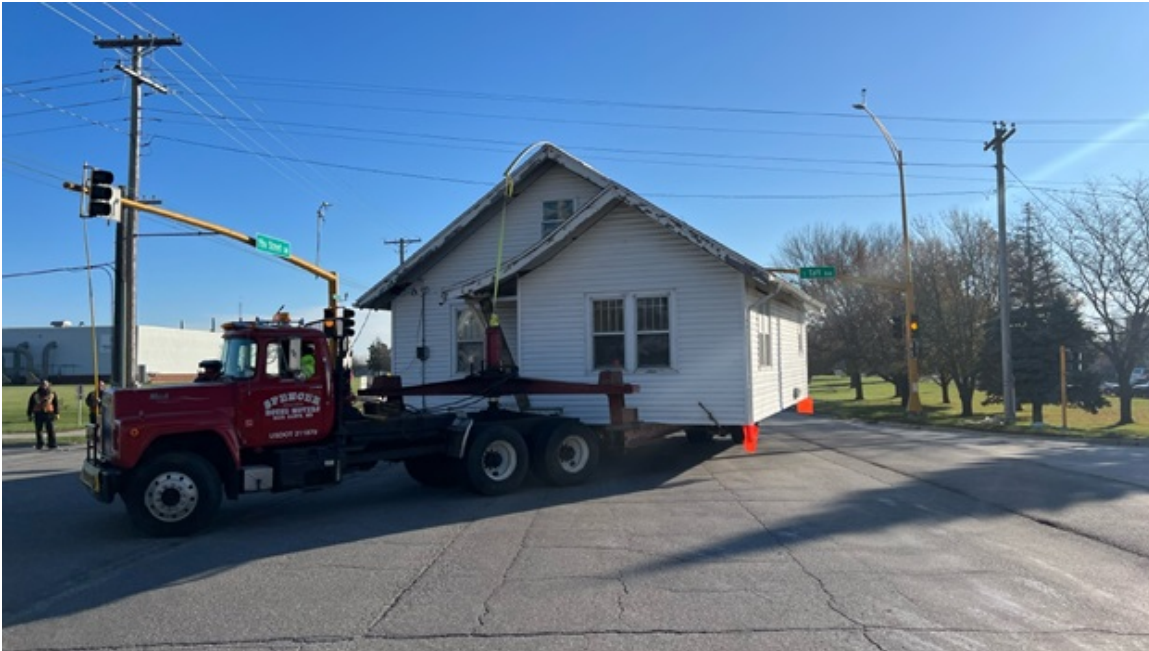
House Move from Blackmore Site to 1526 South Taft Avenue- November 2023
