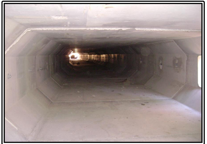
Mason Creek Culvert
